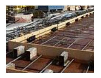
3. Pulling anchors for post-tensioning cables
