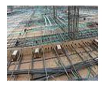
6. Positioned posttensioning cables
