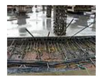
8. Post-tensioning cable ends extending from concrete slab
